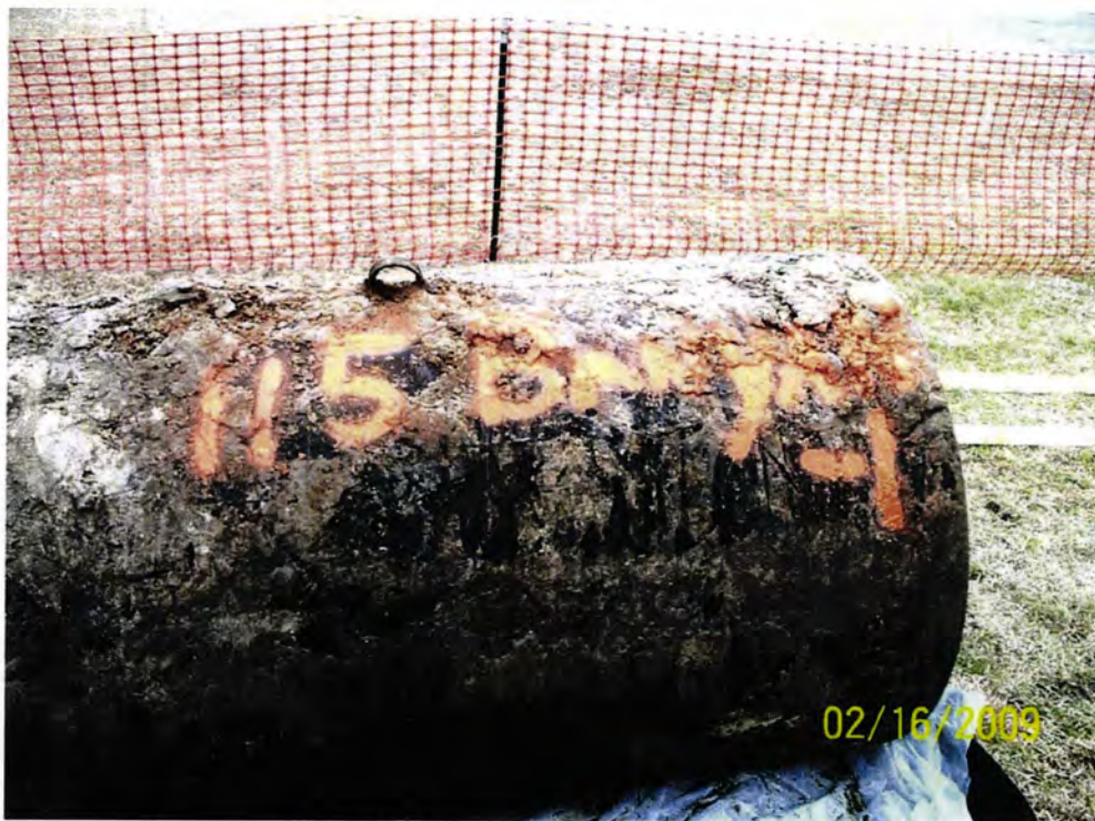
Picture 2: UST 115 Banyon-1 UST prior to cutting for scrap.
